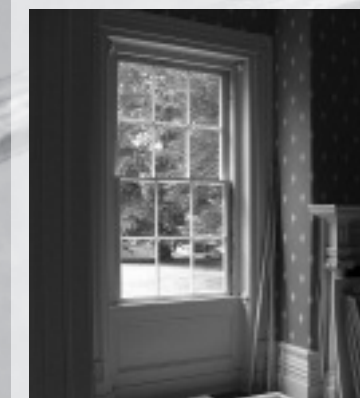
Newly installed window in Orlando Brown House. OB fanlight as background.
